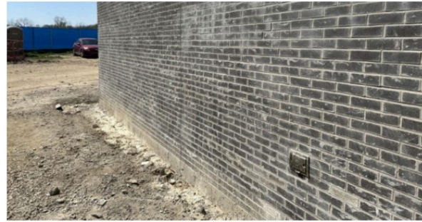
Exterior: building masonry in-progress
