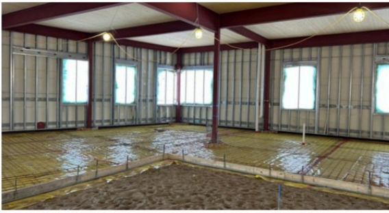
Interior: vapor barrier installation in-progress
