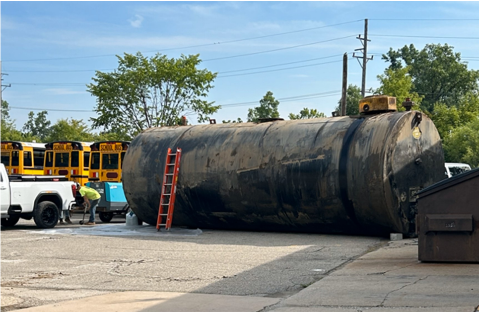
Transportation Center - Underground Fuel Tank Removal
