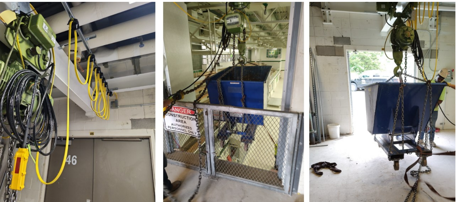
Huron High School - Pool Monorail System to Service Pool Deck and Pool Mechanical Room
