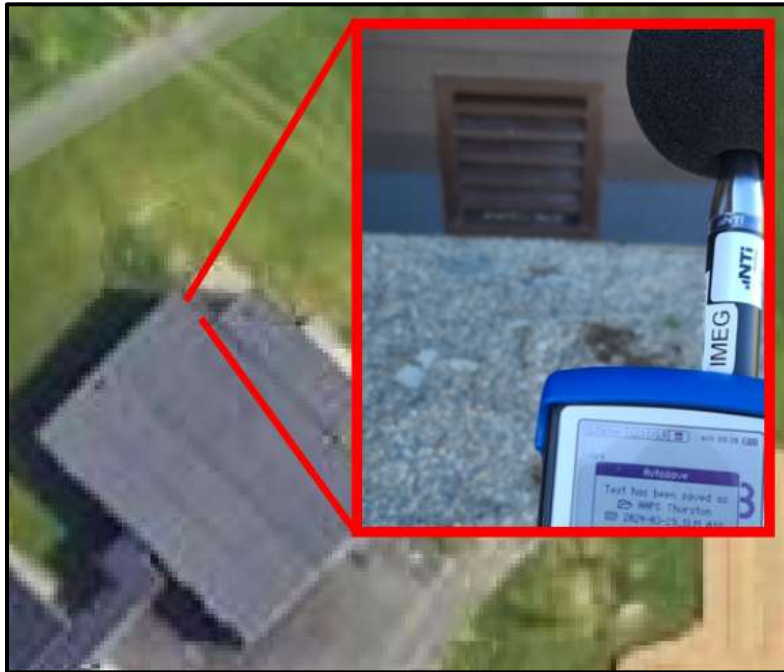
Figure 6: First Loud Exhaust Louvres
