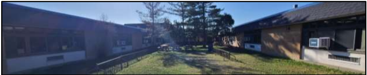
Figure 2: Courtyard with Air Conditioning Units in Every Classroom
