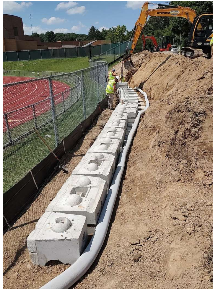
Huron High School - Retaining Wall between Track and Driveway
