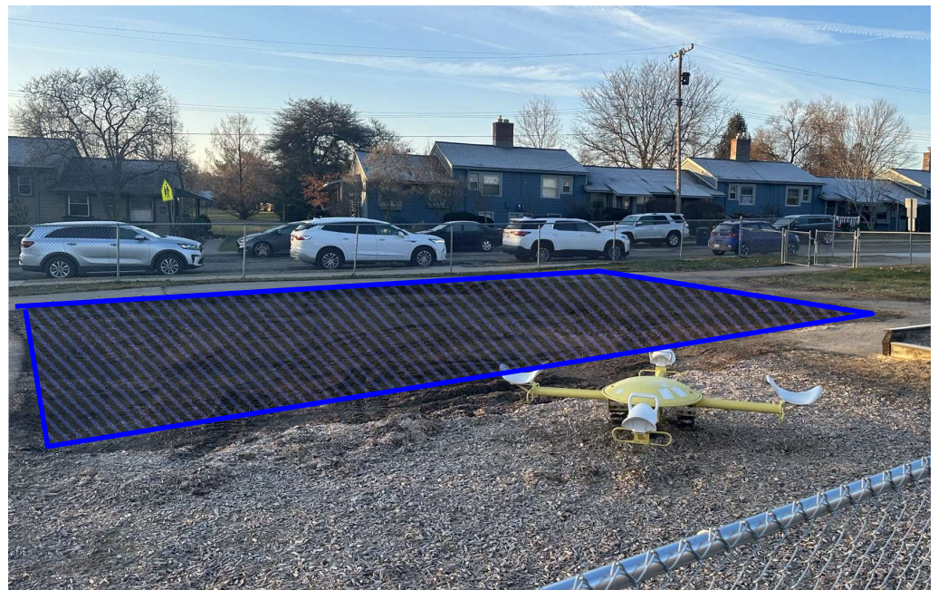
Pittsfield Elementary - Excavation for New Preschool Playground (in process)
