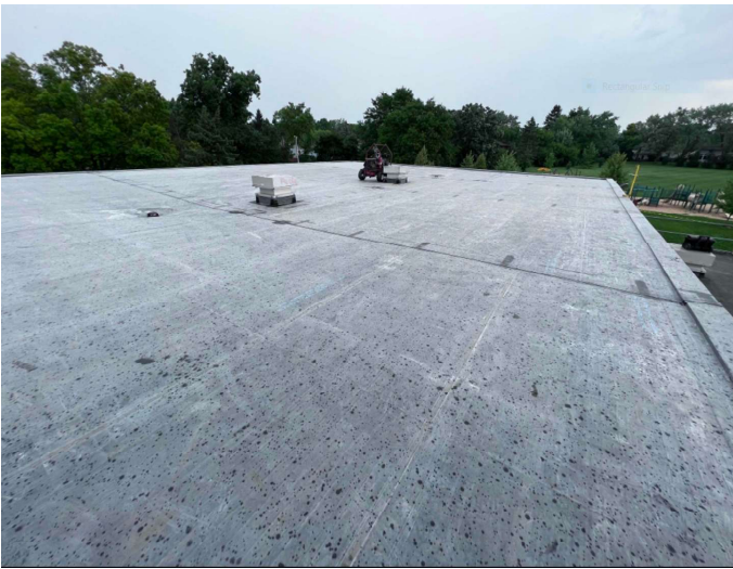
Abbot Elementary School – Roofing Improvements
