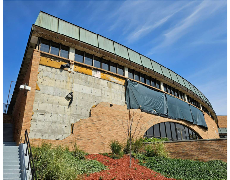
Huron High School - Emergency Brick Repair
