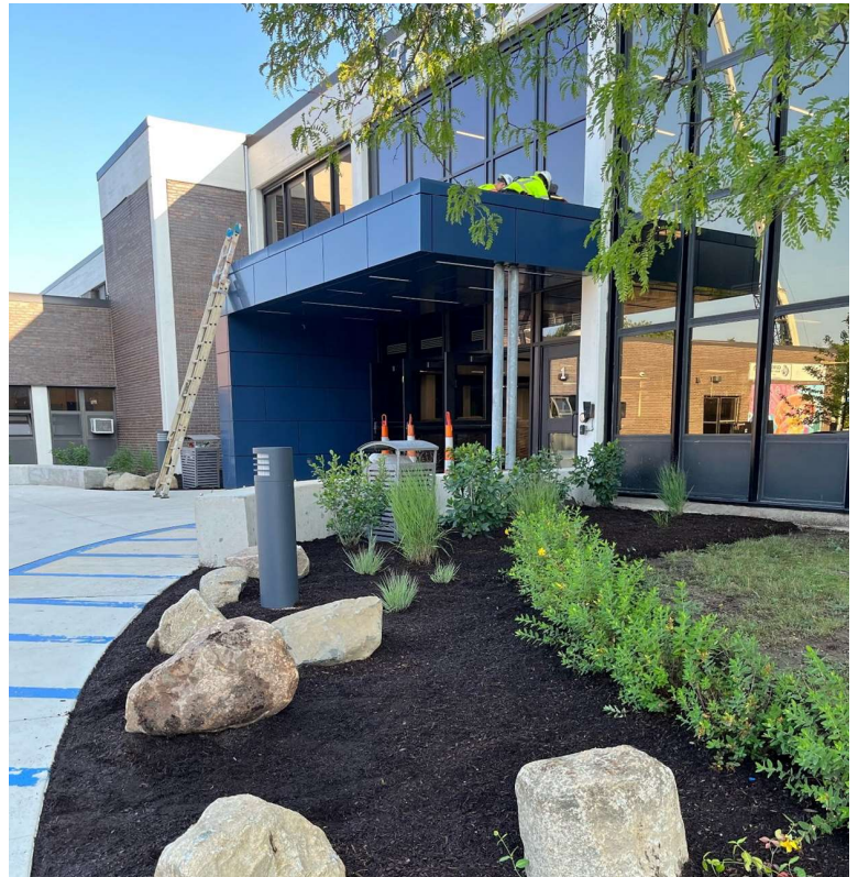
New Front Entrance and Canopy
