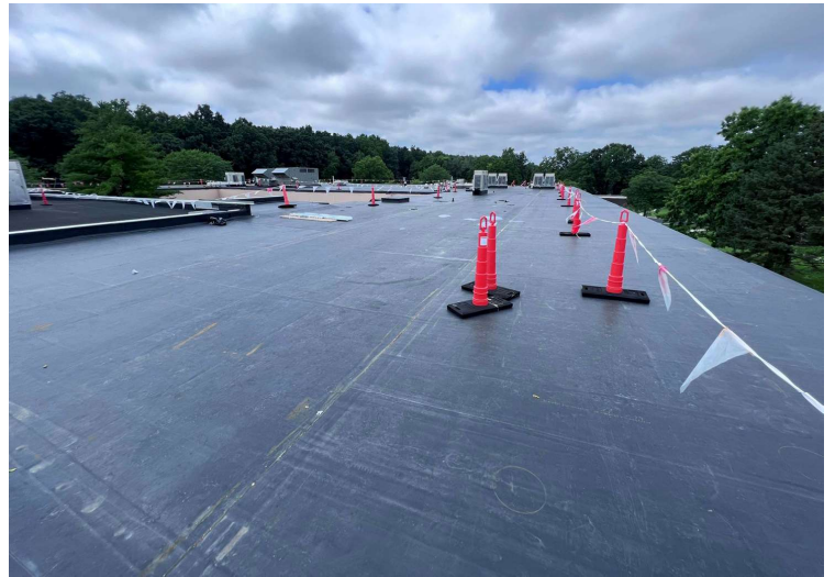
Scarlett Middle School - Roof Replacement
