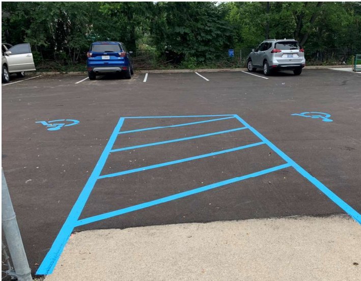
Bach Elementary - Parking Lot Paving
