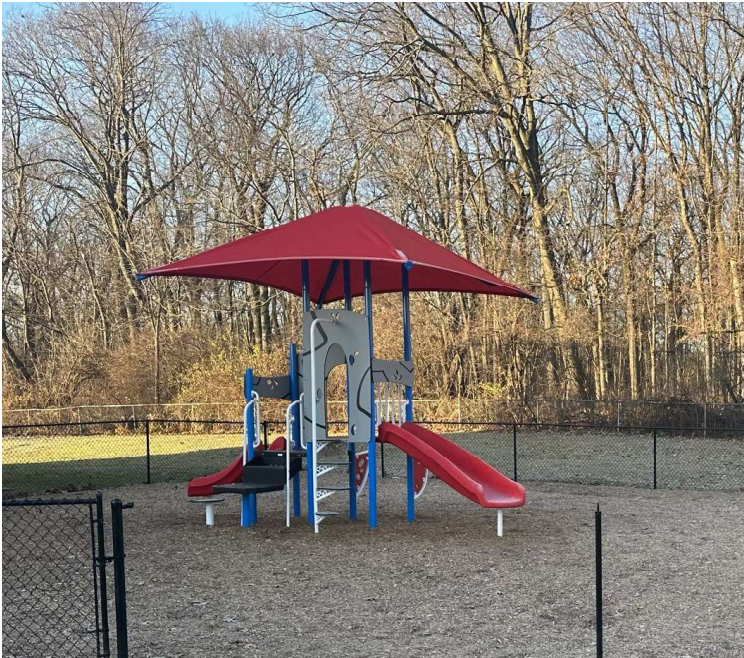
Lakewood Elementary - New Preschool Playground (in process)
