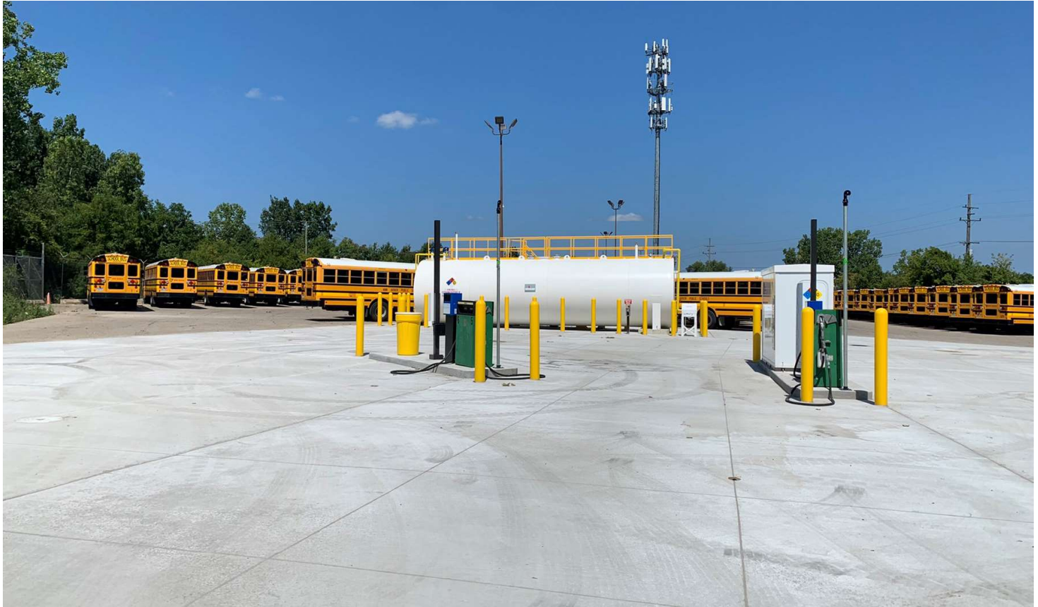
Transportation Center - Fuel System Improvements
