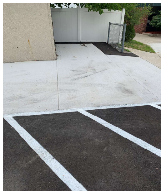
Bach Elementary - Parking Lot Paving
