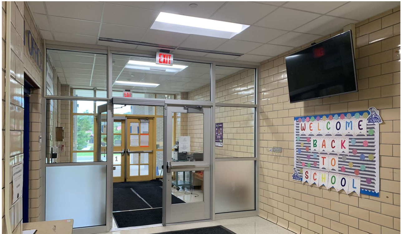
Tappan Middle School - New Vestibule at Main Entrance
