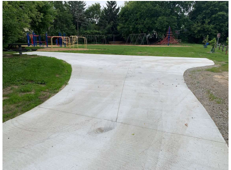
Bach Elementary - Paved Entrance to Playground
