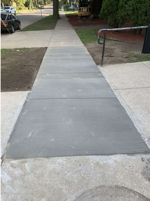
Bach Elementary - Storm Water Pipe Replacement
