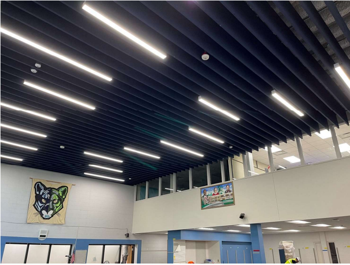
Media Center LED Lighting & New Acoustic Ceiling
