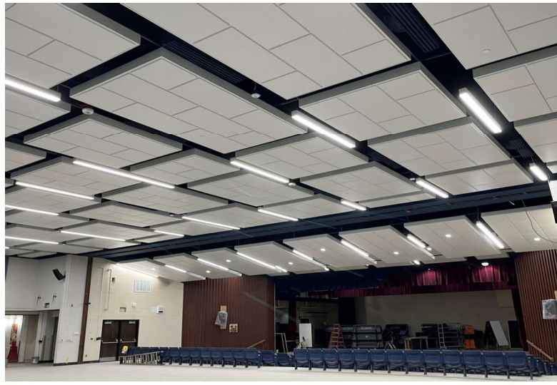
Multi-purpose Room LED Lighting & New Acoustic Ceiling
