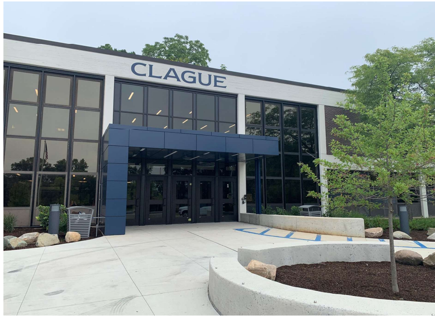
New Front Entry with Canopy
