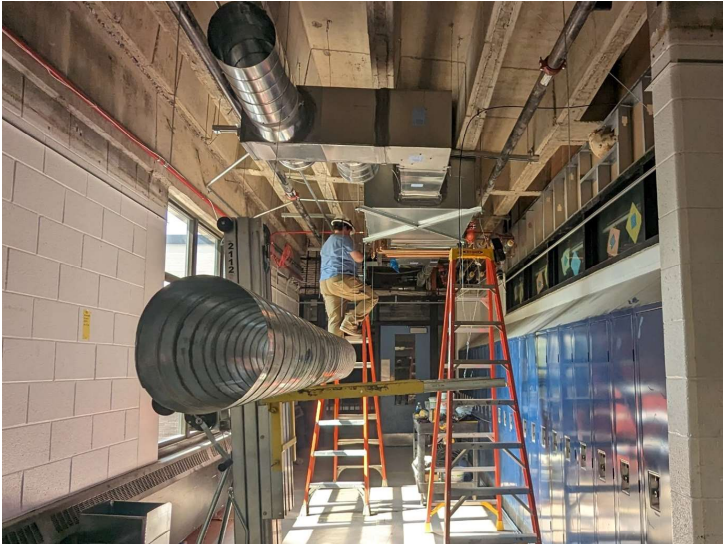
New Mechanical Ductwork
