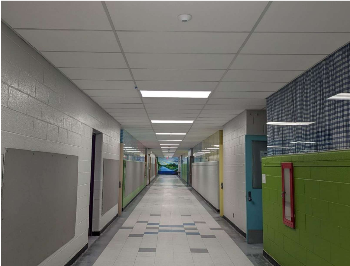
Wines Elementary School – Air Conditioning, LED Lighting, and Ceiling Replacement
