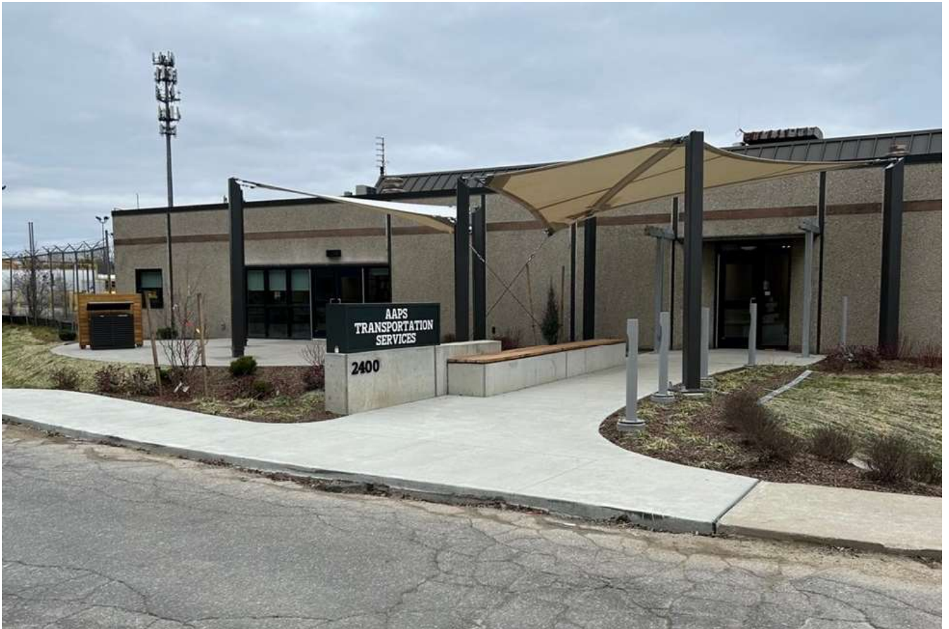
Transportation Center - New Entrance
