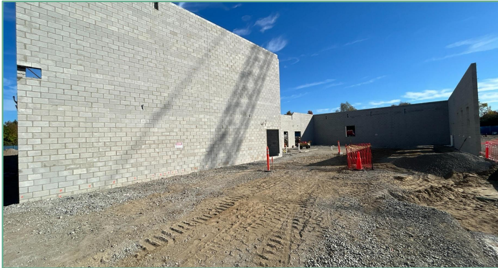
Unit A Masonry: Kitchen and Servery Exterior Walls Complete
