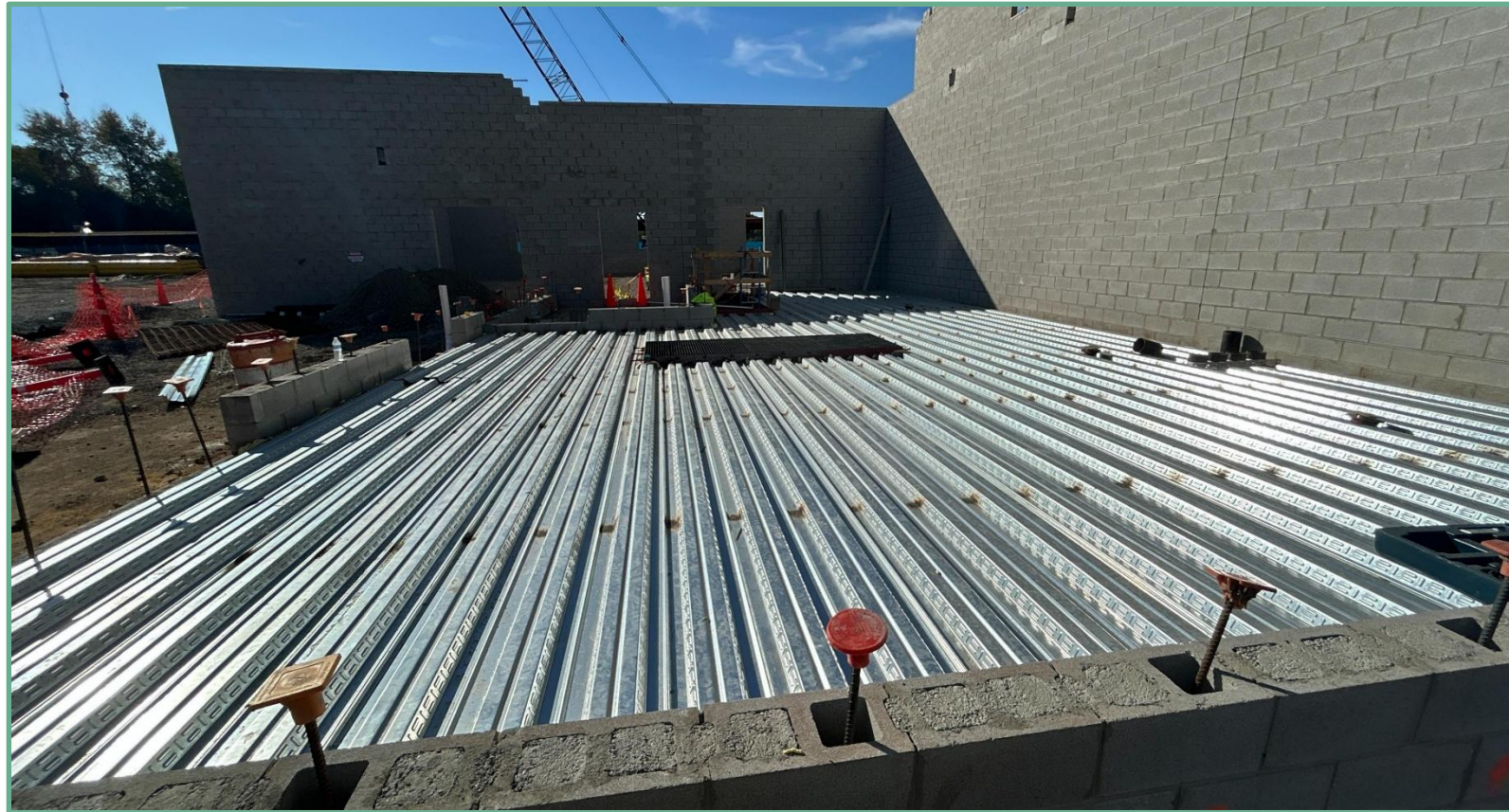
Unit A: Steel Deck Installed at Mechanical Vault
