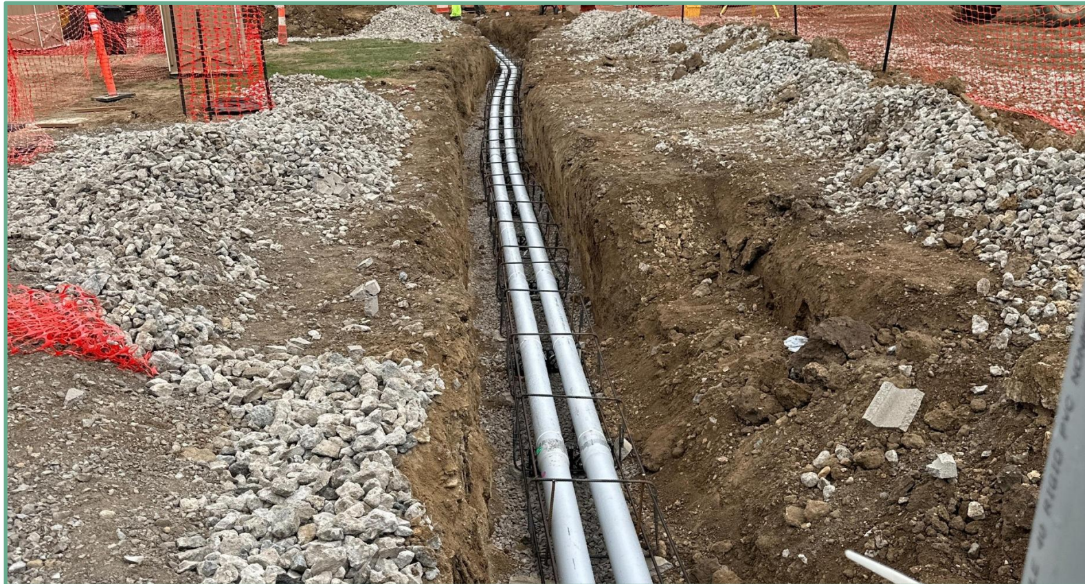
Site: Installing DTE feed to building
