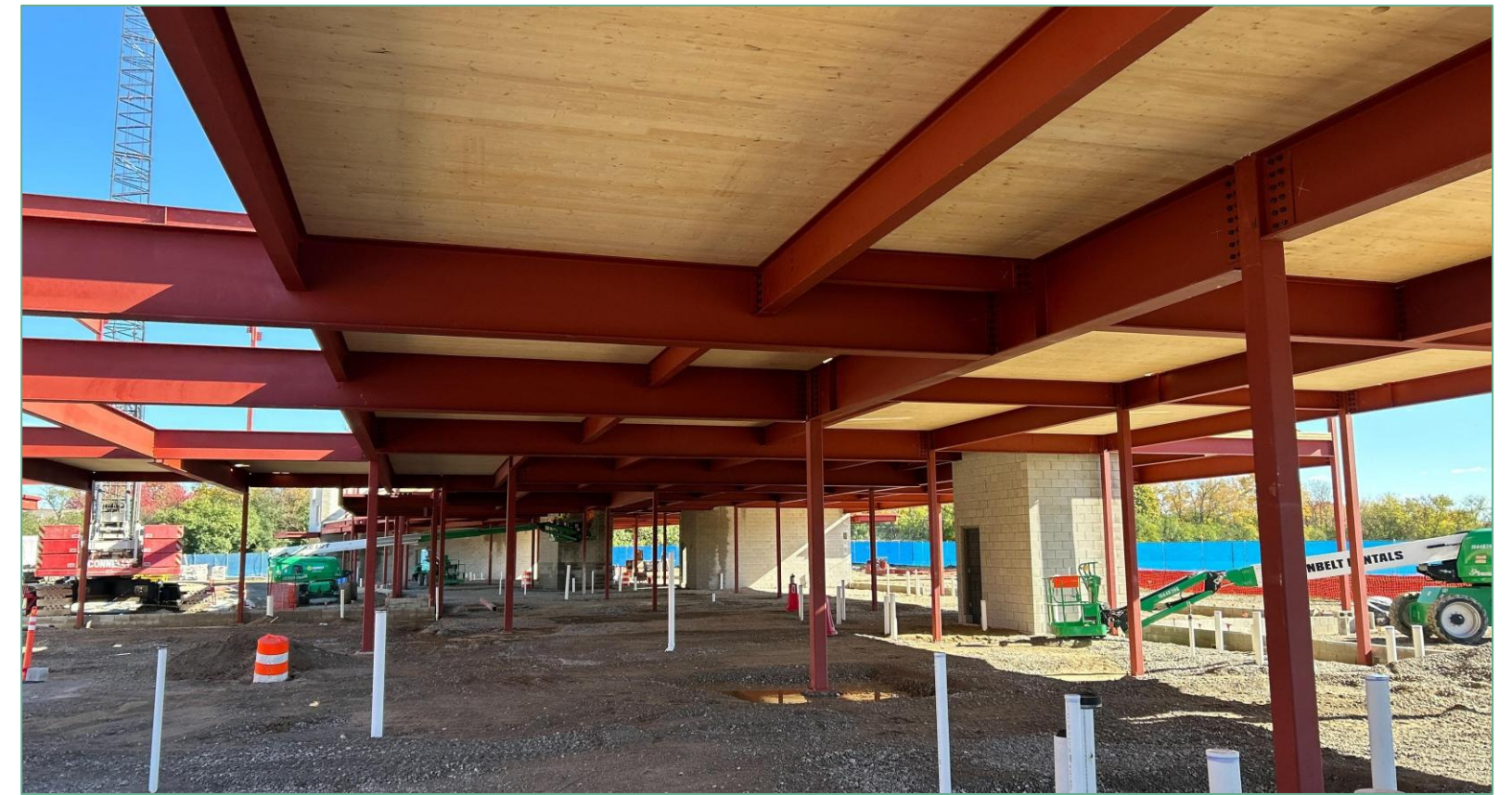
Unit B: Setting CLT on Second Floor
