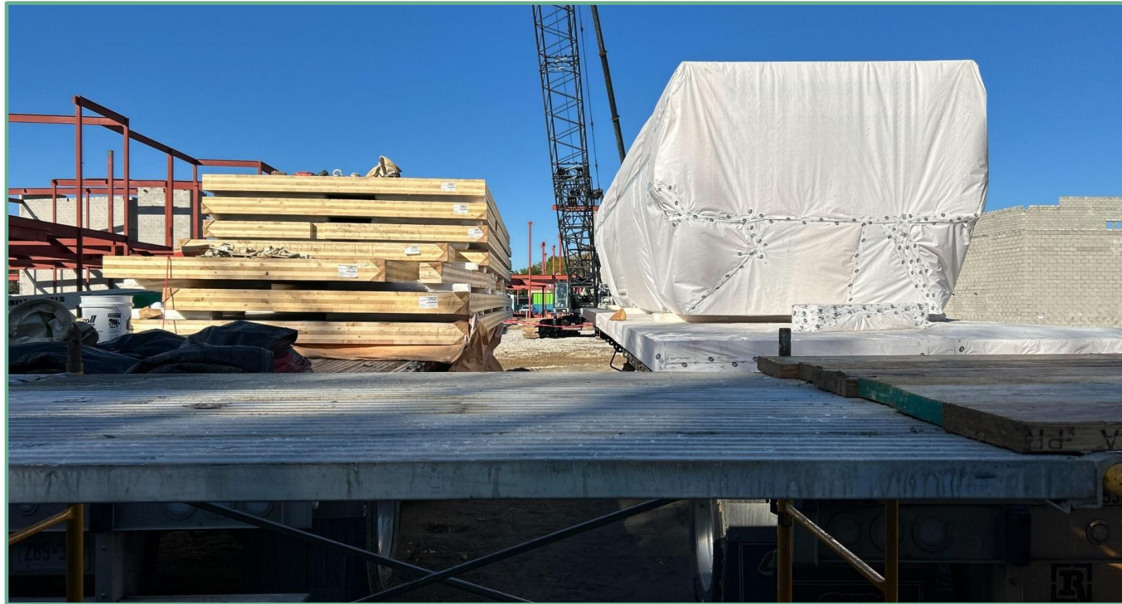
Unit C: CLT Delivery and Staging
