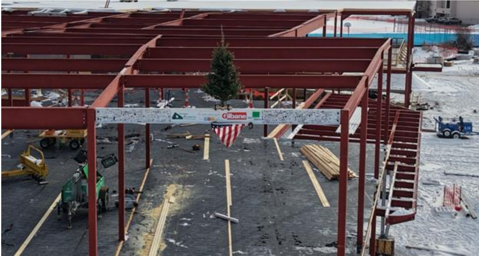
Steel Topping Out 12/03/25
