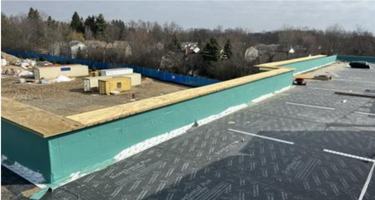
Roof Parapet Cap & Waterproofing Installation
