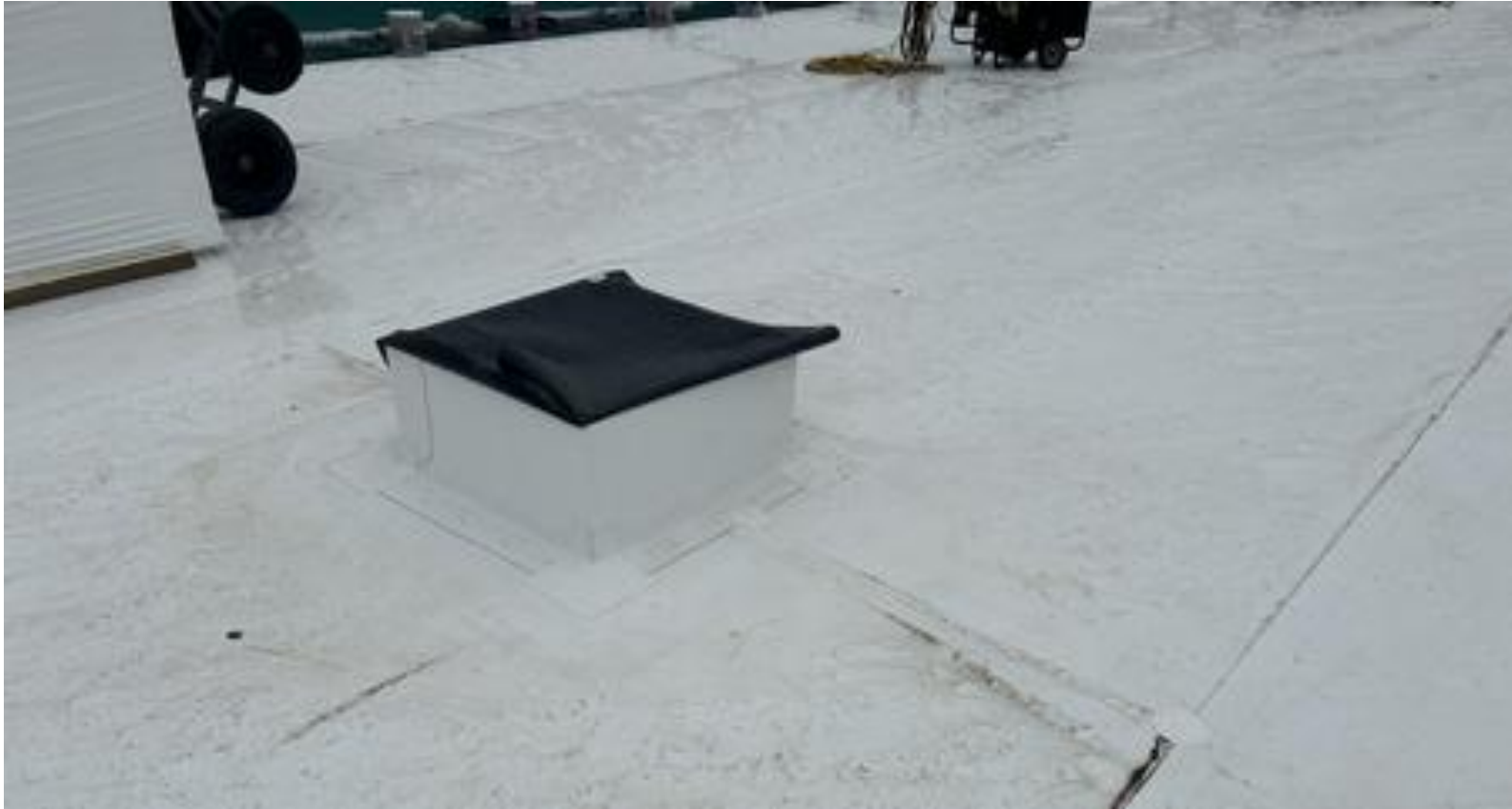
Roof Curbs & Insulation with Roofing Membrane
