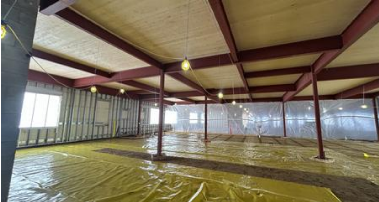
Vapor Barrier in Classrooms
