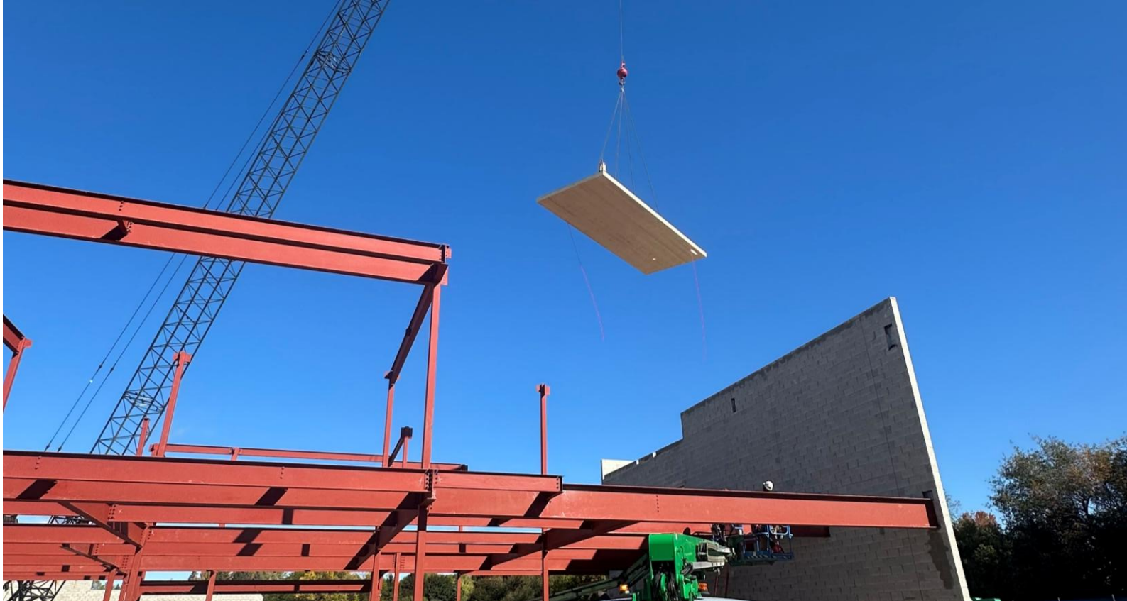
CLT Lift and Placement
